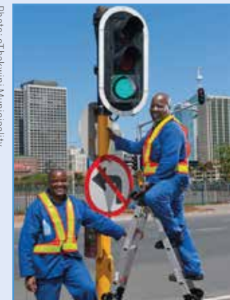
Replacing traffic lights with energy efficient LEDs
