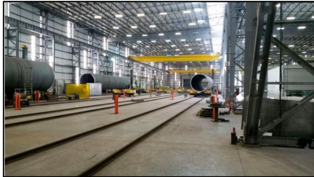
FIGURE 8: DCD WIND TOWERS, PORT ELIZABETH
